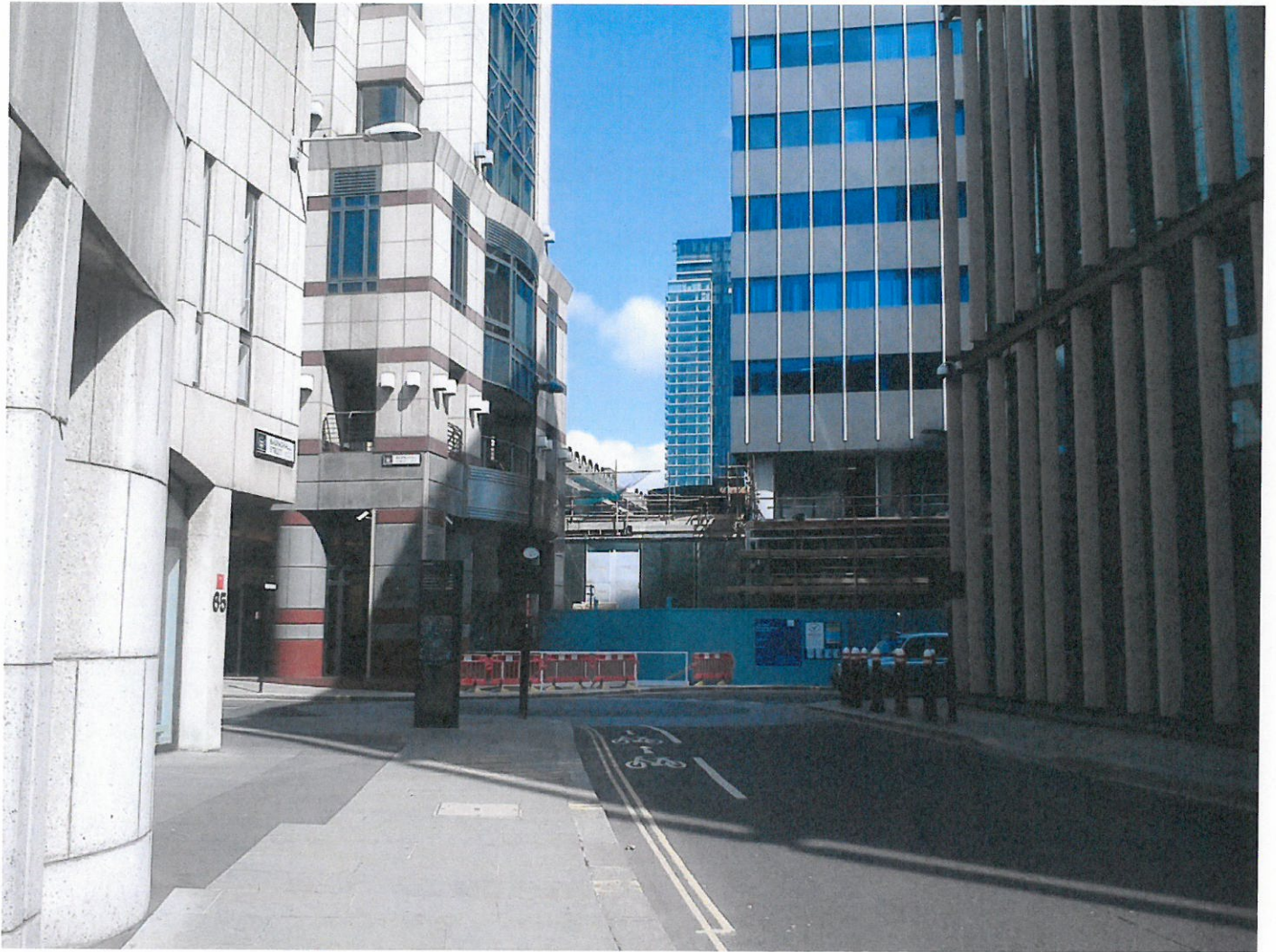
View from Basinghall Street
